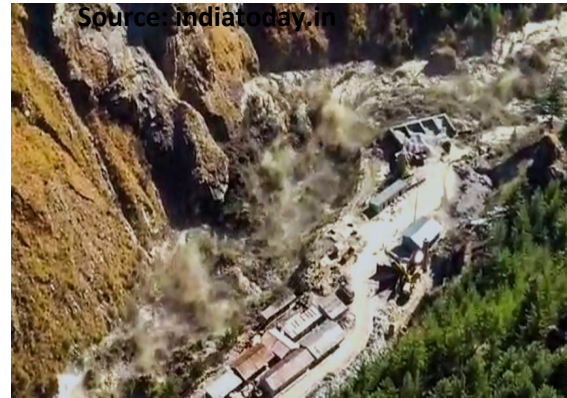
Hydropower plant in Uttarakhand damaged by the flash floods
